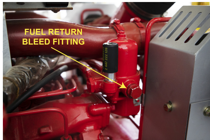
FIGURE 23 - FUEL RETURN LINE CONNECTION
