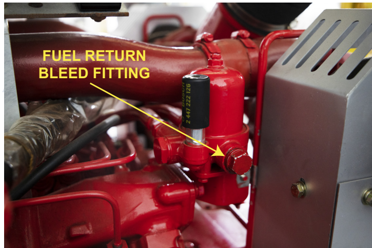
FIGURE 23 - FUEL RETURN LINE CONNECTION
