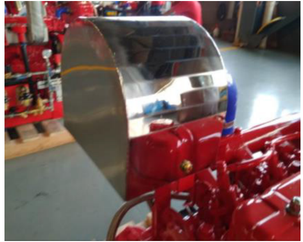
FIGURE 19 - AIR FILTER HOUSING
