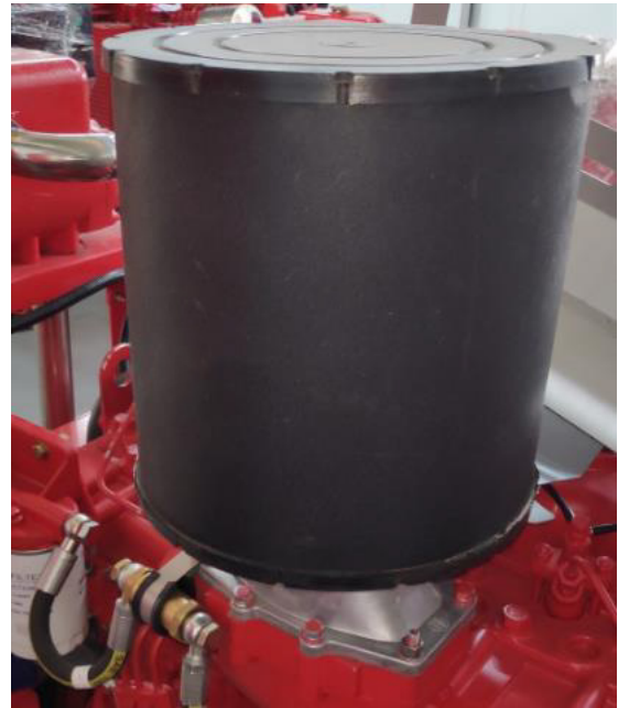
FIGURE 19 - AIR FILTER HOUSING
